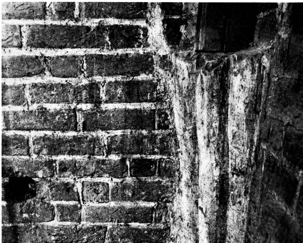
Fig. 86. Hvælvrest i nordre korsarms nordøstre hjørne (p. 206). - Remains of vaulting in the north-east corner of the north transept.
