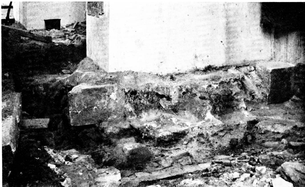
Fig. 36. Sondering i søndre koromgang ved anden pille fra korsskæringen (p. 139). — Probe in the south ambulatory near the second pier from the crossing.
