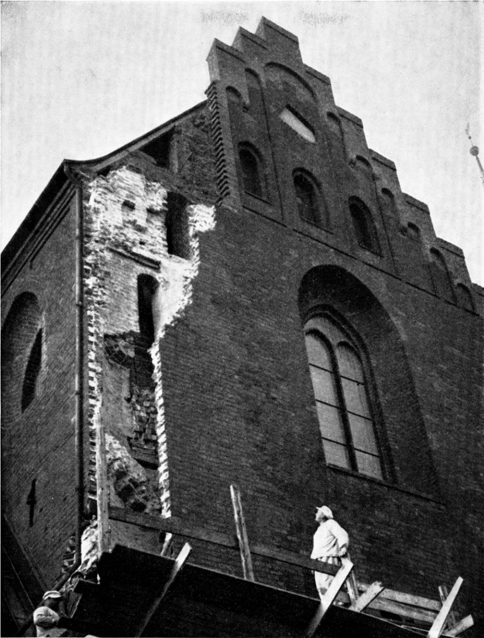
Fig. 57. Nordre korsarms gavl med rester af muret spindeltrappe (p. 163). — The end wall and gable of the north transept with remains of brick-built newel stair.
