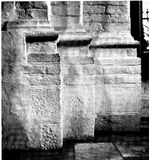
Fig. 43. Nordøstre korsskæringspille, søndre del af vestsidens sokkelparti (p. 144—45). — North-east pier at the intersection of nave and transept, south part of the plinth on the west side.
