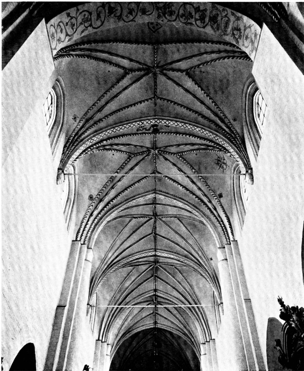
Fig 110. Midtskibets hvælvzone, set mod vest. — The vaulting of the nave, looking west,
