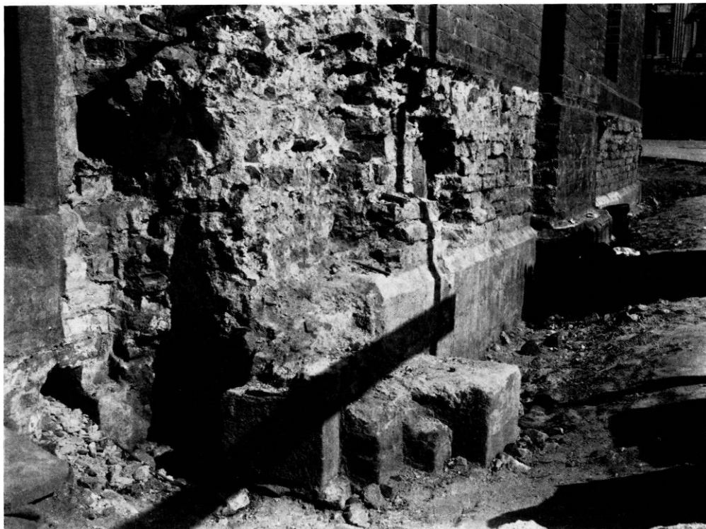
Fig. 50. Søndre korsarms portal, rester af det østre fremspring afdækket 1922 (p. 153). — The portal of the south transept, remains of the east projection revealed 1922.
