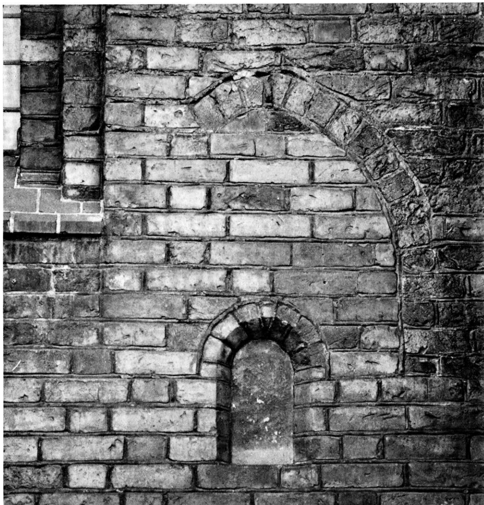
Fig. 93. Tilmurede vinduesåbninger i nordre sideskibs vestligste fag (p. 217). — Walled-up window embrasures in the bay furthest to the west in the north side aisle.
