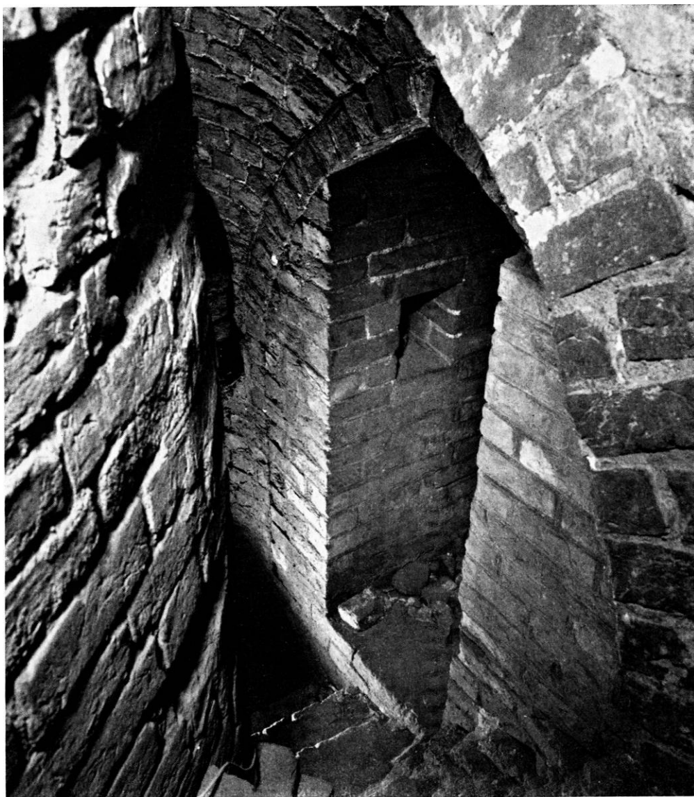
Fig. 128. Tilmuret vindue i hjørnet mellem søndre korsarm og koret (p. 264). — Walled-up window in the corner between the south transept and the choir.
