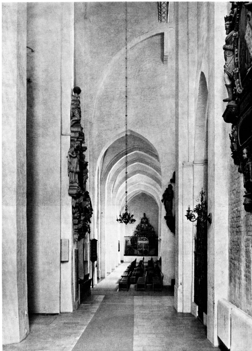
Fig. 89. Nordre koromgang og nordre sideskib, set mod vest. — North ambulatory and north side aisle, looking west.
