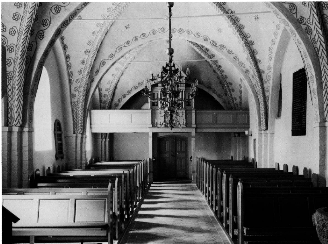
Fig. 9. Indre, set mod vest. NE fot. 1977. - Interior looking west,
