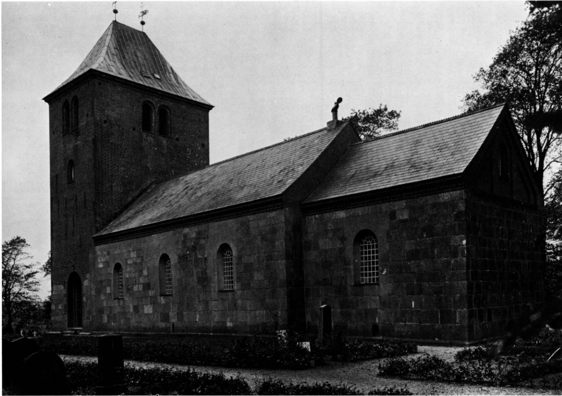
Fig.7. Kirken set fra sydøst. Victor Hermansen fot. 1934. - The church seen from south-east.
