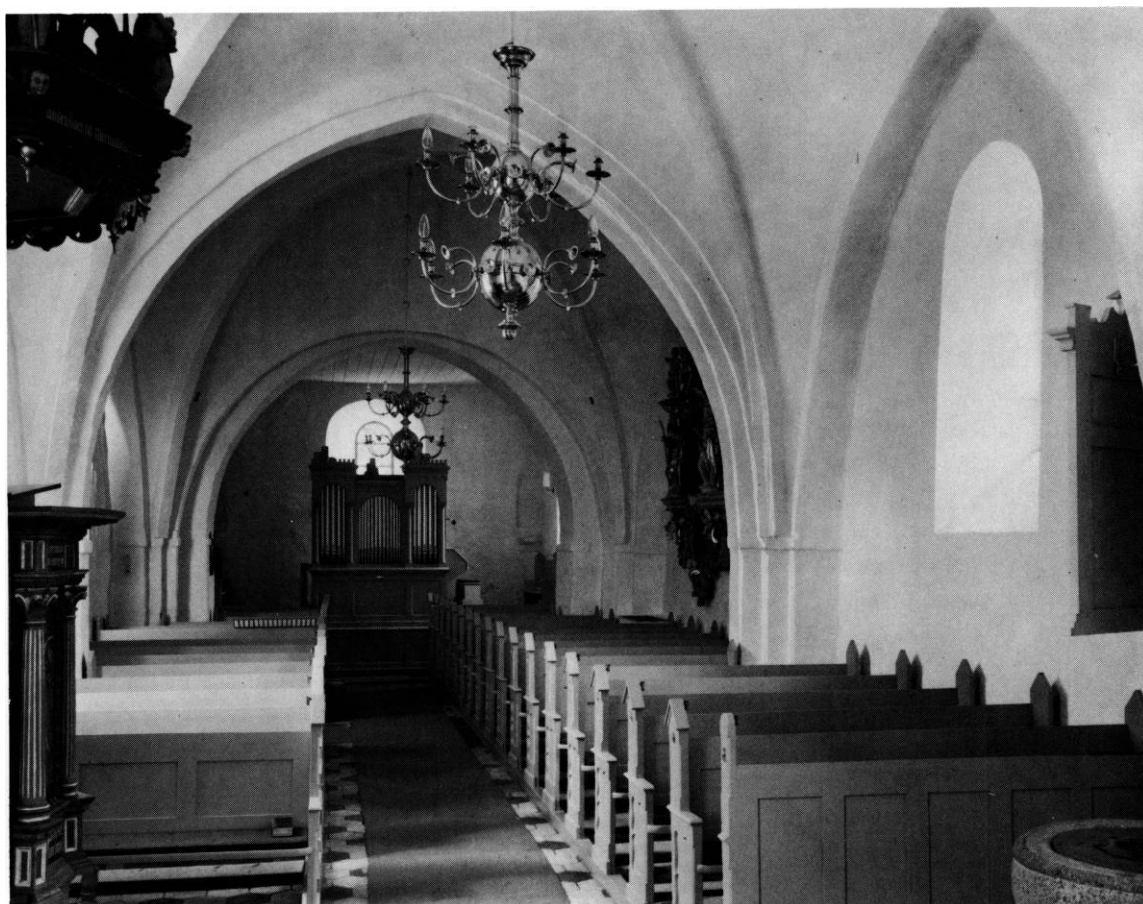
Fig. 10. Indre, set mod vest. NE fot. 1978. - Interior looking west.
