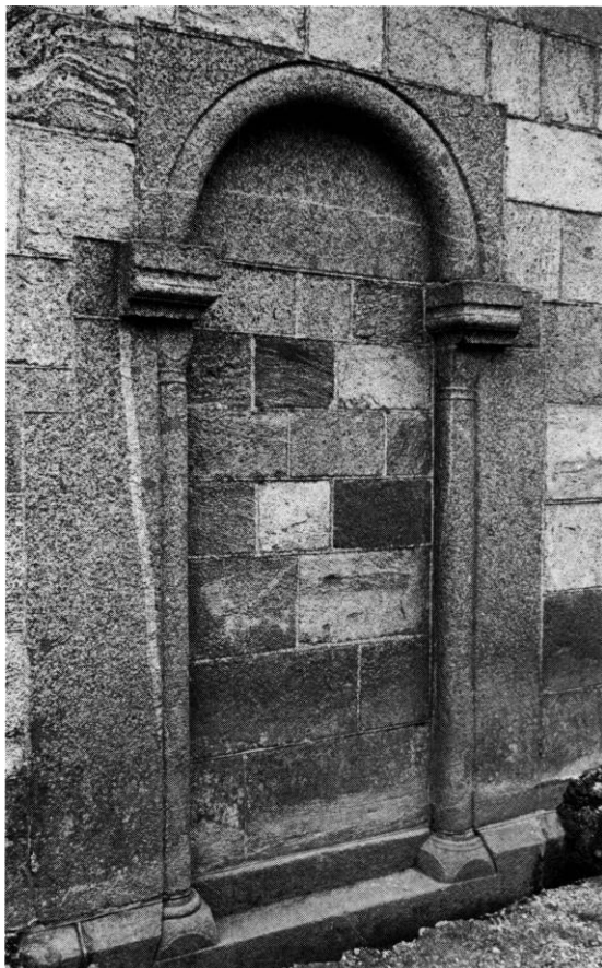
Fig. 5. Tilmuret nordportal (s. 1905) med frigravet sokkel. NJP fot. 1981. - Walled up north doorway with exposed plinth.
