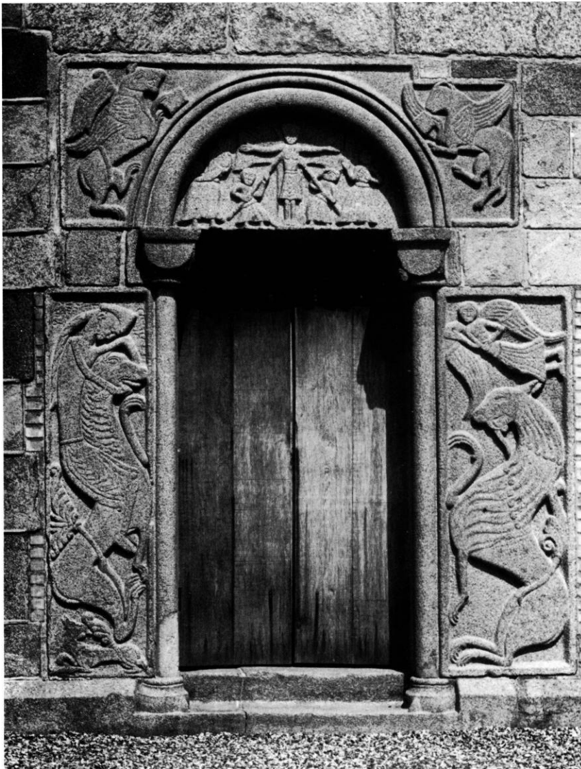
Fig. 7. Granitportal i skibets sydmur (s. 2089). J.J.F. fot. 1979. - Granite portal in south wall of nave.
