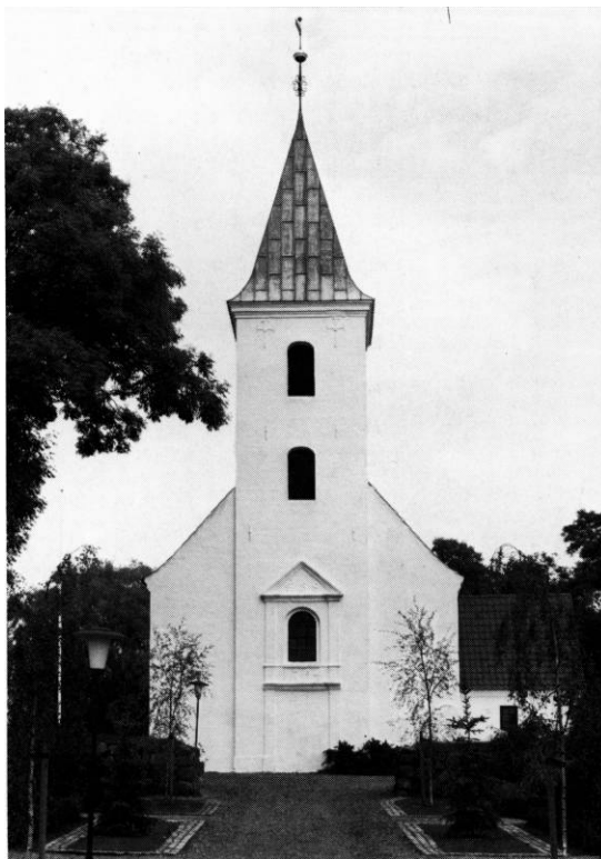
Fig. 7. Kirken set fra vest. NE fot. 1980. - The church seen from the west.
