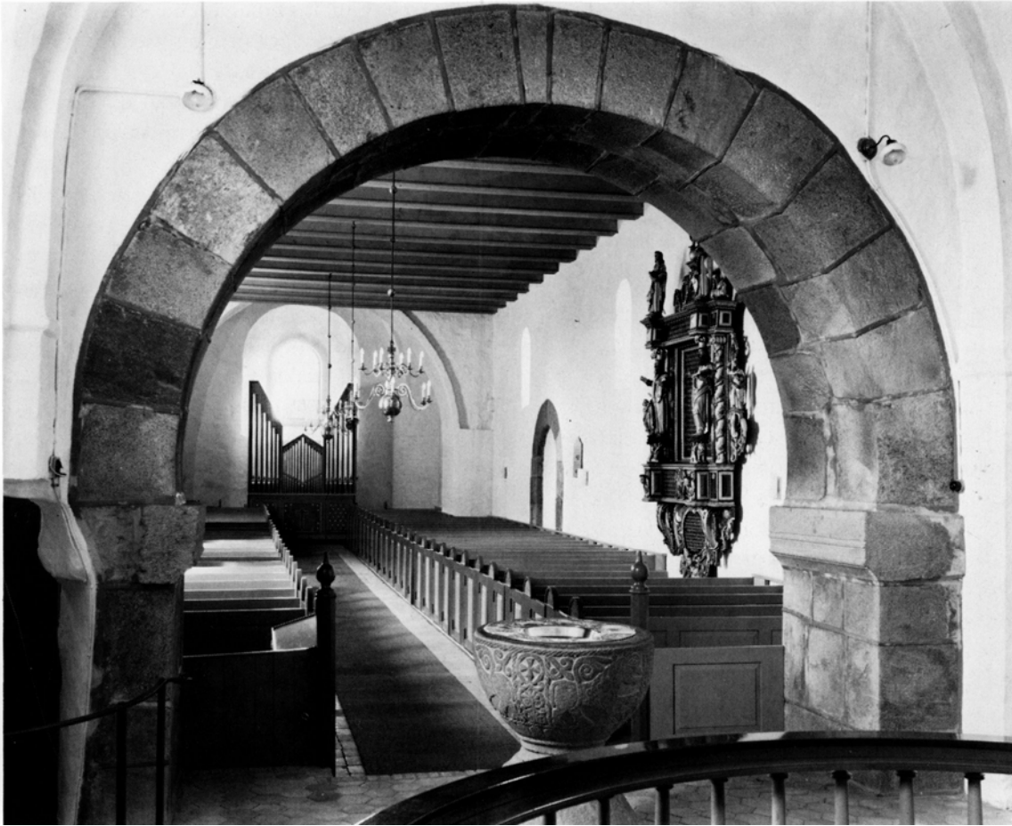
Fig. 32. Indre, set mod vest. NE fot. 1981. - Interior looking west.
