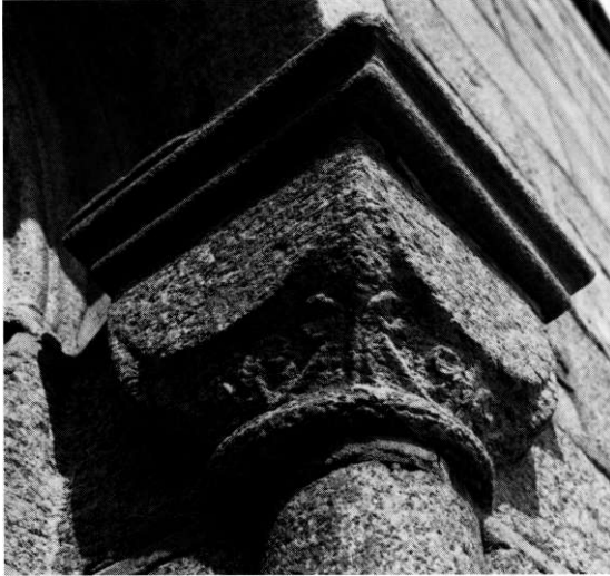
Fig. 11. Østre kapitæl i korportalen (s. 2754). KdeFL fot. 1986. - The capital furthest to the east in the entrance to the chancel.
