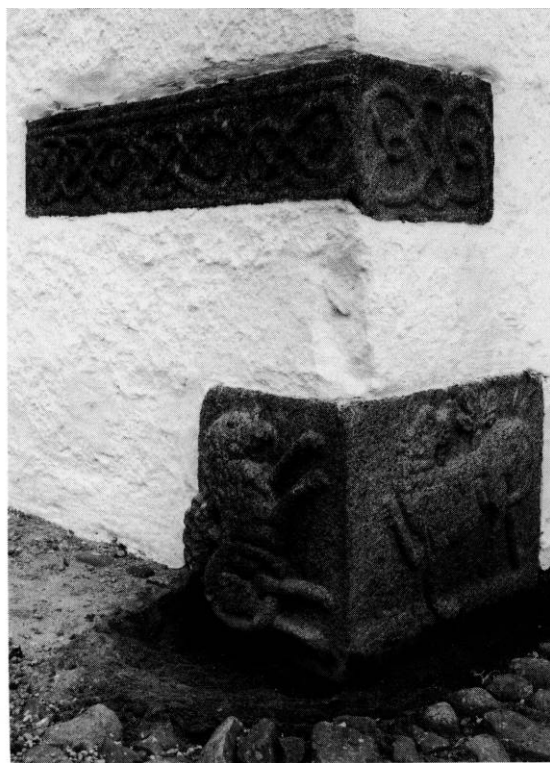
Fig. 11. Reliefkvadre indmuret i kirkens sydvestre hjørne (s. 3024). NE fot. 1984. - Carved ashlar's included in the south-west corner of the church.
