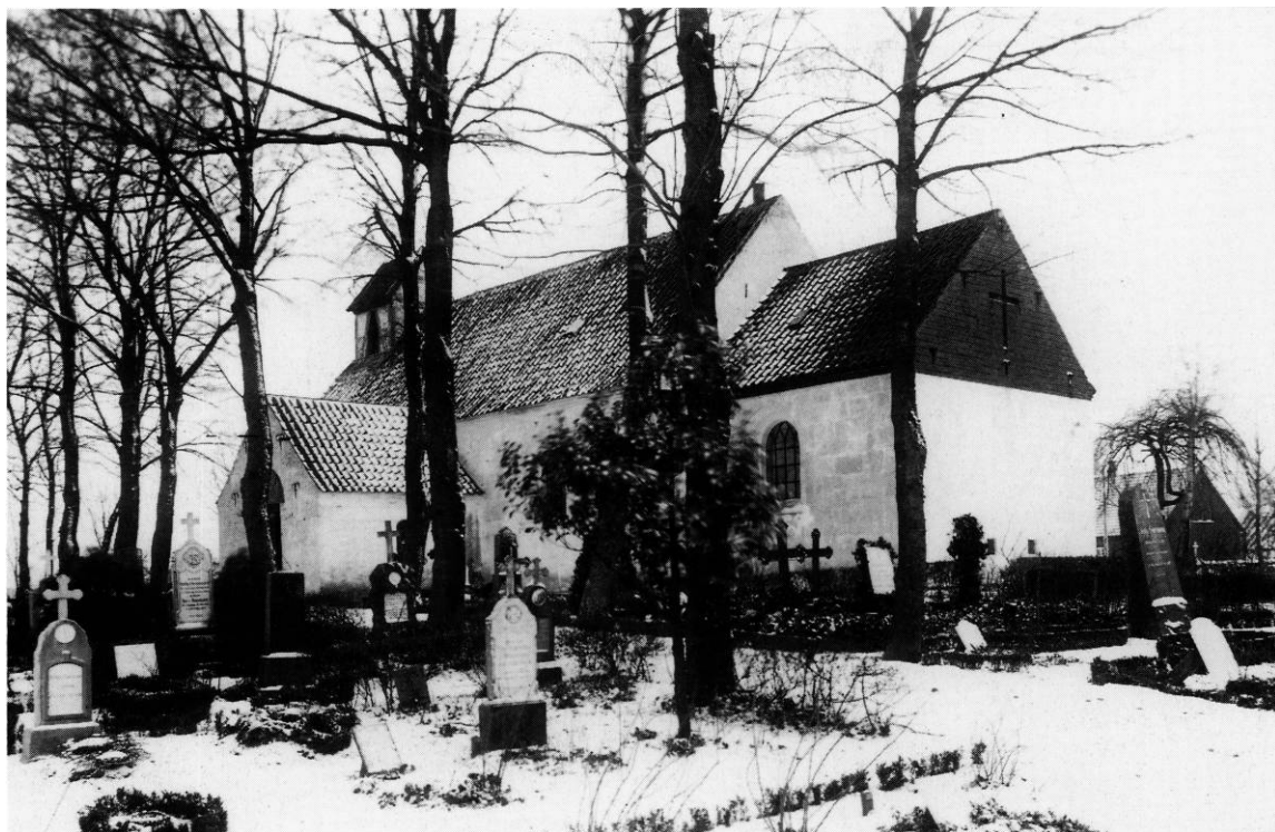
Fig. 3. Kirken set fra sydøst. Foto omkring 1910 i Kgl. Bibl. - The church seen from the south-east.
