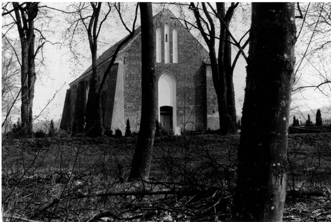
Fig. 11. Kirken set fra nordvest. KdeFL fot. 1990. - The church seen from the north-west.
