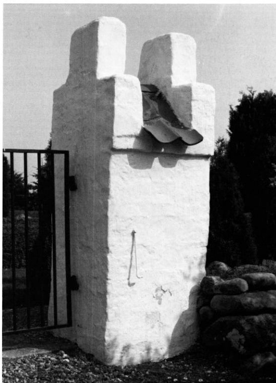
Fig. 2. Kirkegårdsportens søndre pille. KdeFL fot. 1993. - The south pillar of the churchyard gate.
