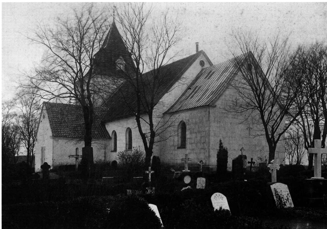
Fig. 45. Kirken set fra sydøst o. 1910. - The church seen from the south-east.
