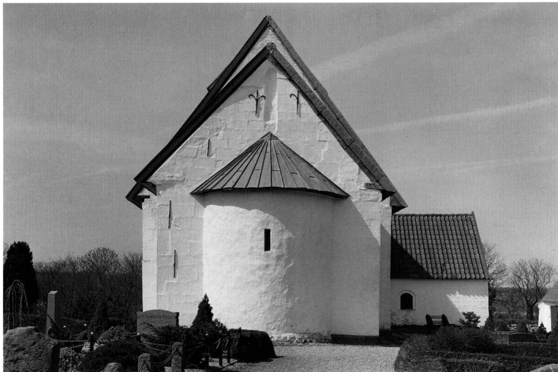
Fig. 10. Kirken set fra øst. KdeFL fot. 1997. - The church seen from the east.
