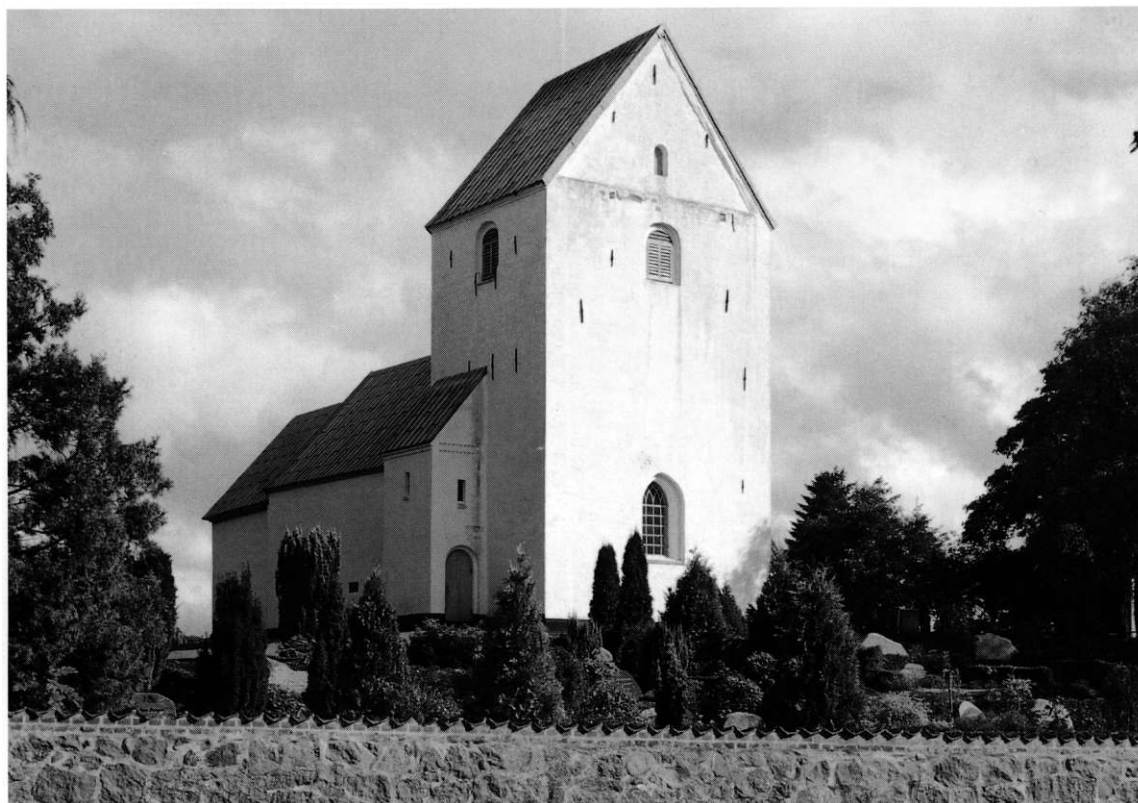
Fig. 1. Kirken set fra nordvest. KdeFL fot. 1997. - The church seen from the north-west.
