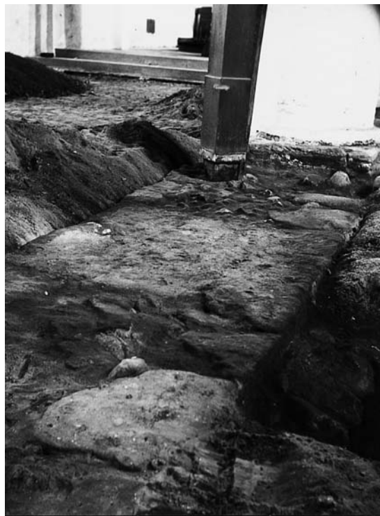
Fig. 50. Udgravning i langhuset 1933. Fremdraget er midtskibets søndre strækmur under 2. arkade, set fra vest. Det lyse felt i midten er aftrykket af en plint, der har båret den fjernede pille (s. 5081f.). Viggo Norn fot. 1933. – Excavation in the nave, 1933. The southern wall section from the central aisle below the second arcade, seen from the west, has been uncovered. The light area in the middle is the impression of a plinth that bore the removed pillar.
