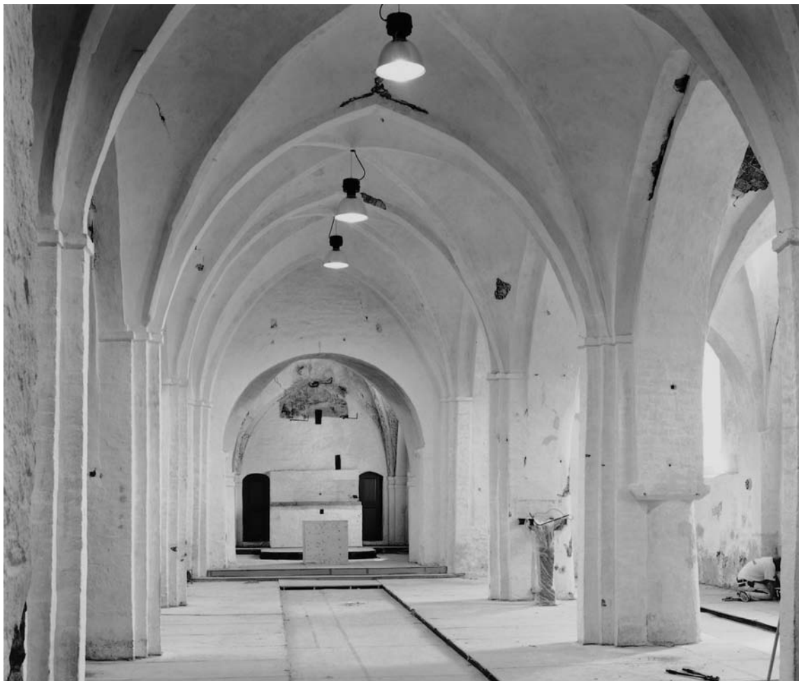
Fig. 45. Indre set mod øst under restaurering. Jesper Weng fot. 2001. – Interior looking east during restoration.
