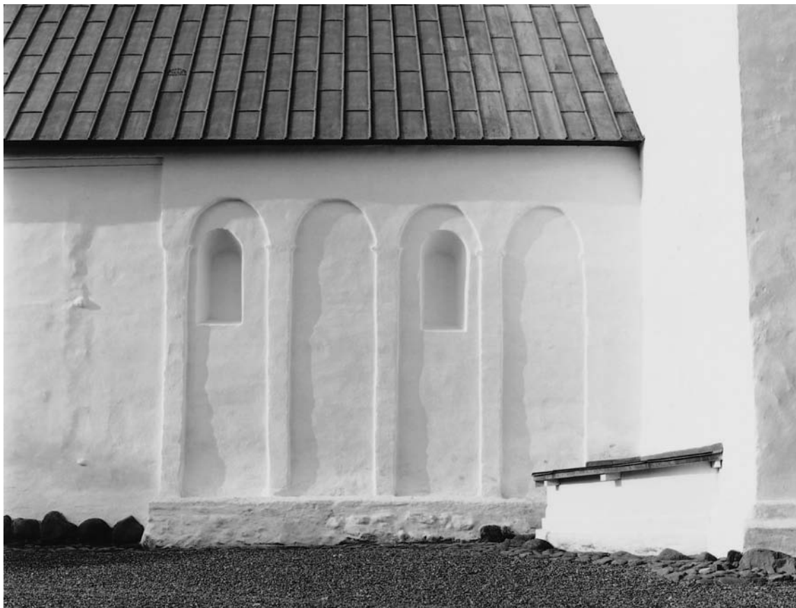
Fig. 26. Korets nordside med facadeudsmykning (s. 5068) og th. langhusets nordre apsis (s. 5071). Jesper Weng fot. 2001. – North side of the chancel with facade decoration and (right) the north apse of the old nave.
