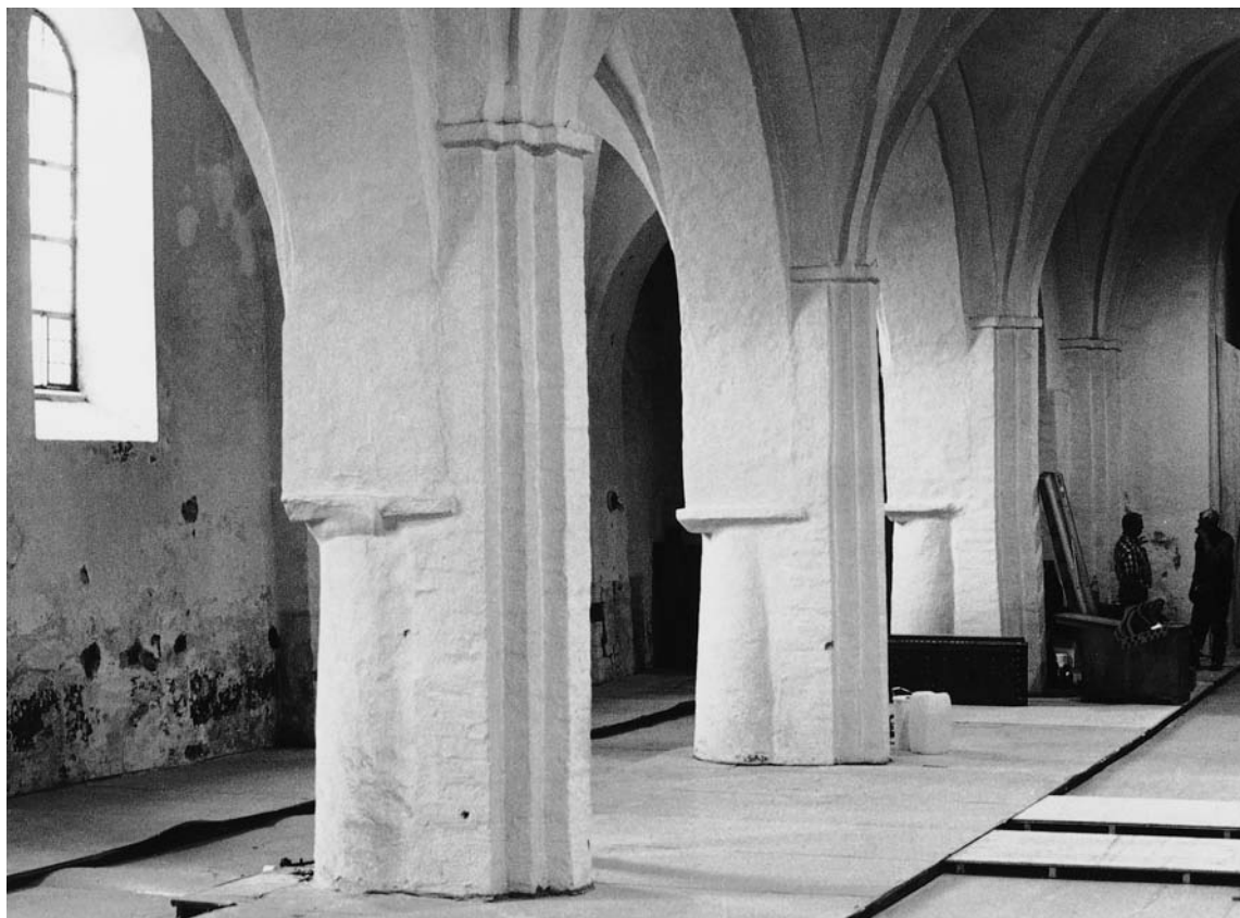
Fig. 39. Langhusets søndre arkademur set mod vest under restaurering. Niels Jørgen Poulsen fot. 2001. – South arcade wall of nave looking west during restoration.
