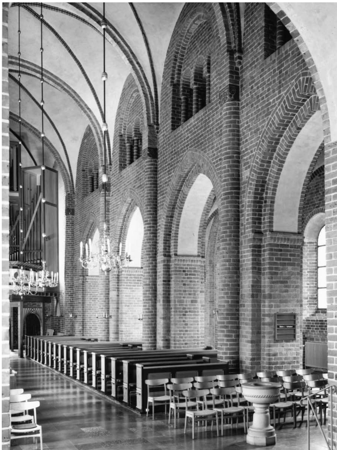
Fig. 119. Nordre midtskibsvæg set fra korbuen. Henrik Wichmann fot. 2002. — North nave wall viewed from the chancel arch.
