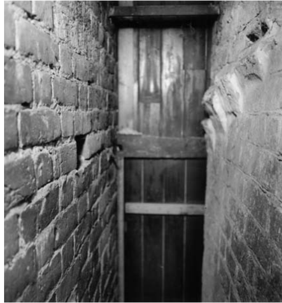
Fig. 65. (†)Ligeløbstrappe i skibets vestgavl med spor af afbrudt loftshvælv, set mod nord (s. 5435). HJ fot. 2003. – (†)Straight-run stair in west gable of nave with traces of broken-off vaulted ceiling, viewed towards the north.
