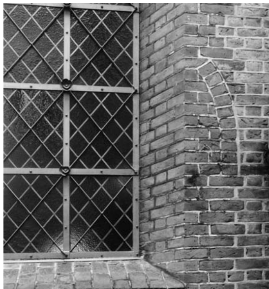
Fig. 43. Detalje af stik fra †dør i nordre sideskibs 4. fag (s. 5417). HJ fot. 2002. – Detail of relieving arch from †door in the fourth bay of the north side aisle.
