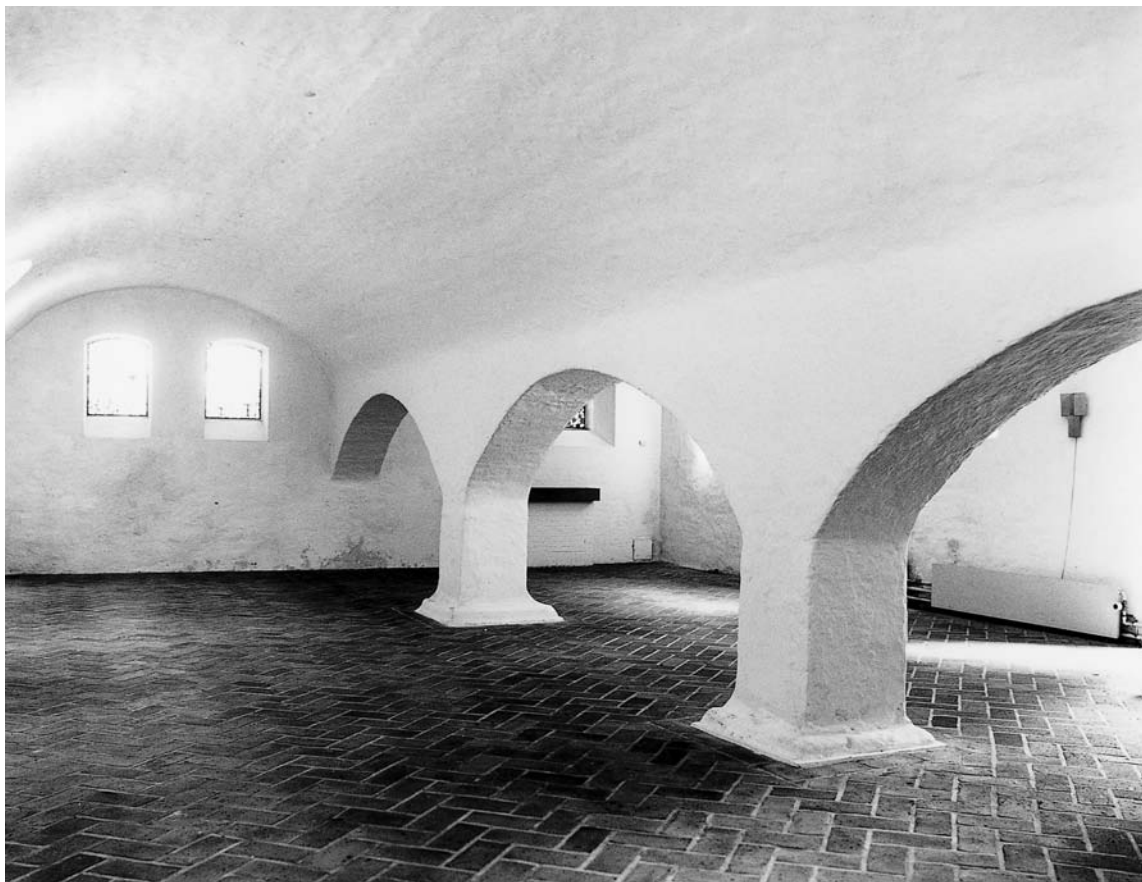
Fig. 25. Kældrens indre set mod nordøst. Foto Roberto Fortuna 2003. – Interior of the basement viewed towards the north east.
