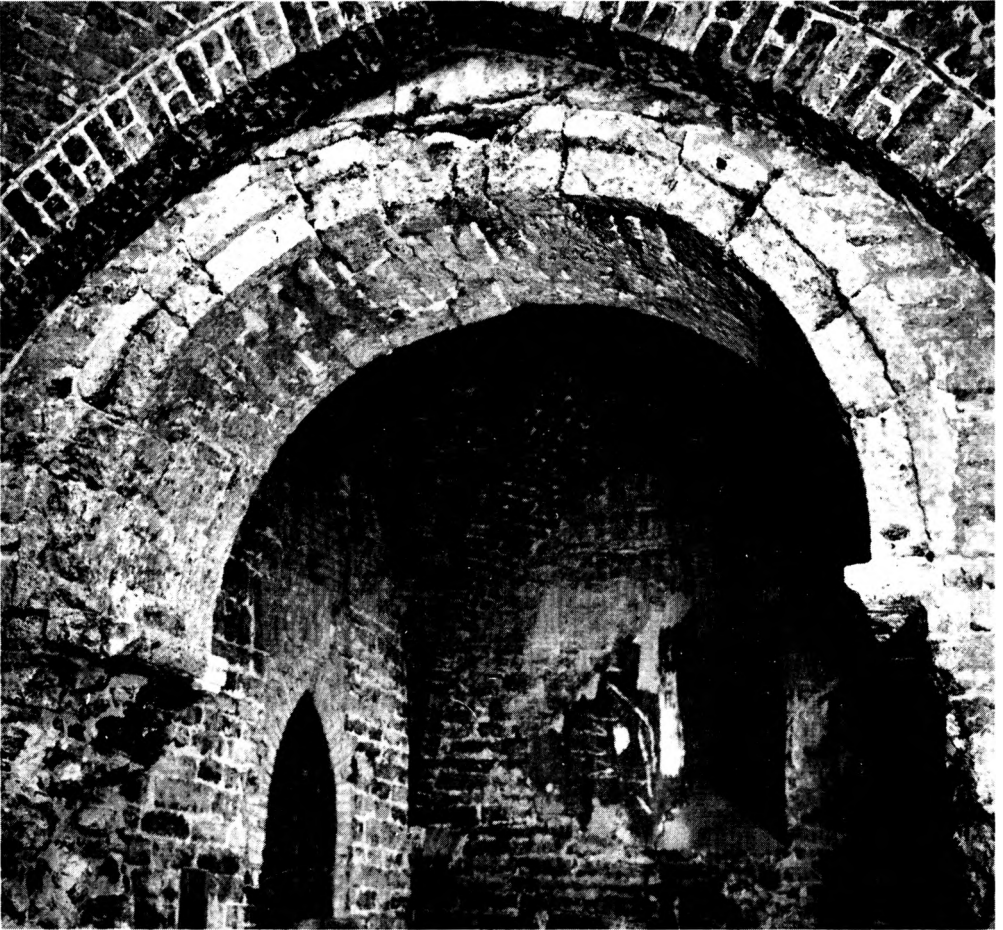
Fig. 4. Krogstrup. Korbuen, set mod øst, under restaurering (p. 2728).
