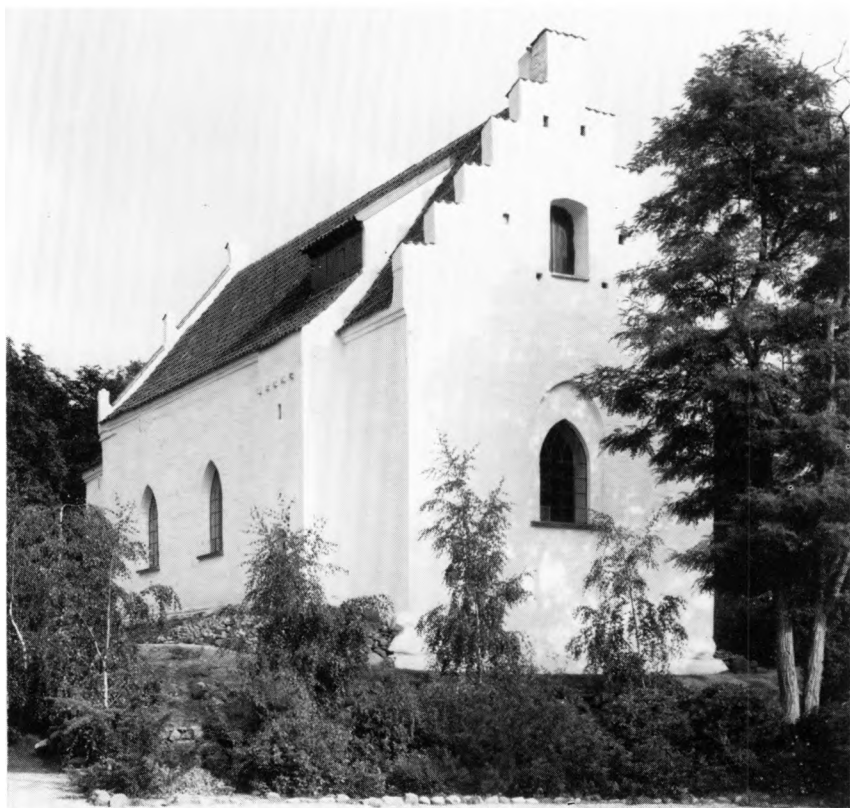
Fig. 6. Ydre, set fra nordvest. LL fot. 1975. — Exterior seen from the north-west.
