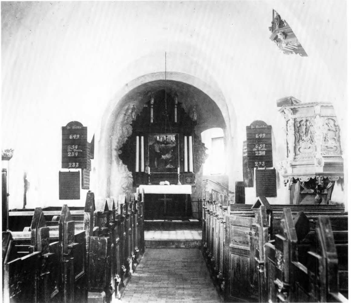
Fig. 10. Indre, set mod øst inden kirkens restaurering 1895. Fot. i NM2. — Interior to the east prior to the church's restoration in 1895.
