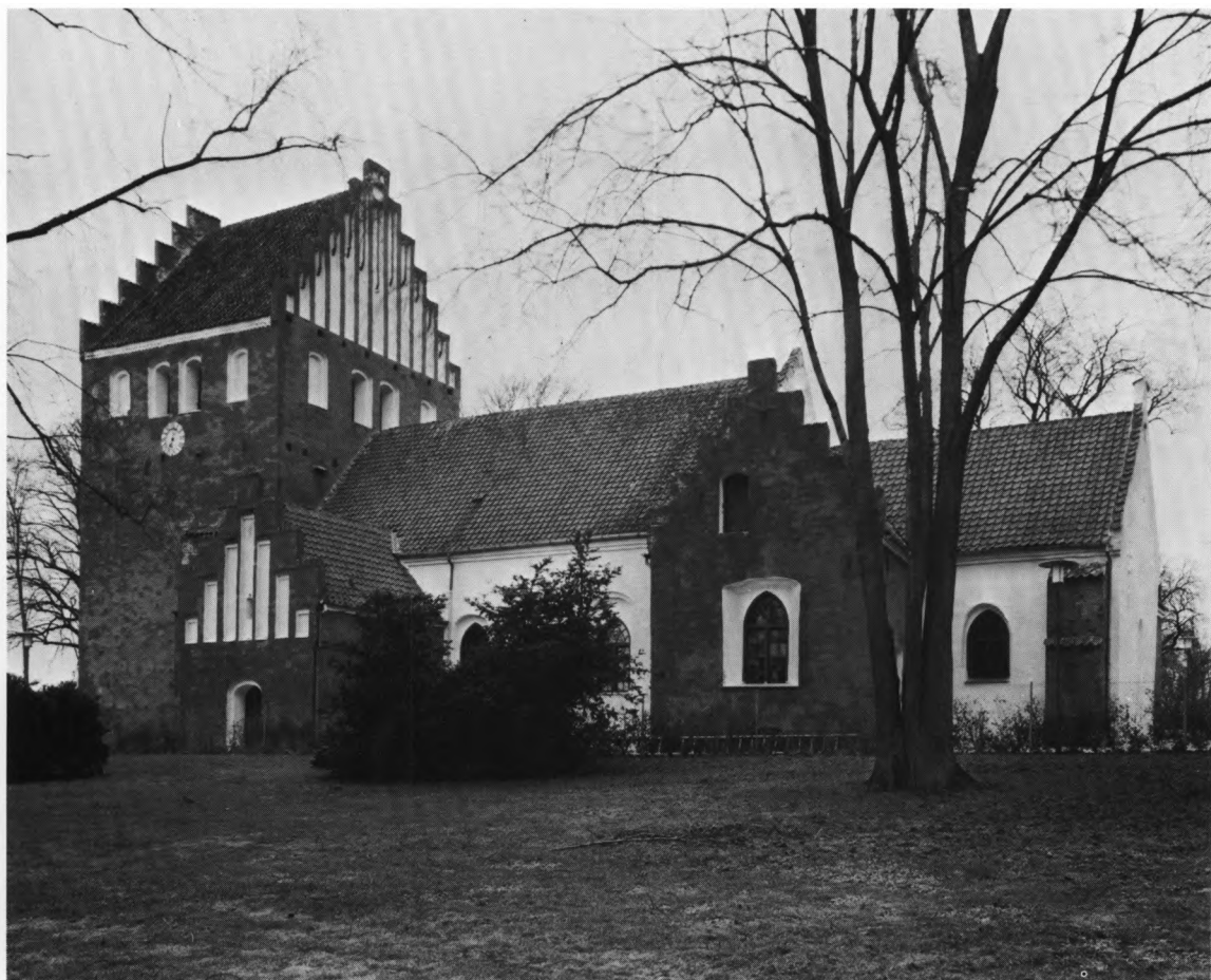
Fig. 8. Ydre, set fra syd. NE fot. 1981. - Exterior seen from the south.
