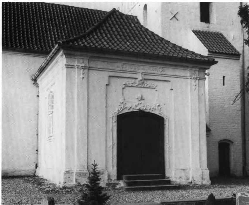
Fig. 6. Gravkapel fra 1769. Facade mod nord (s. 986). HJ fot. 1984. - Mortuary built 1769. Facade to the north.
