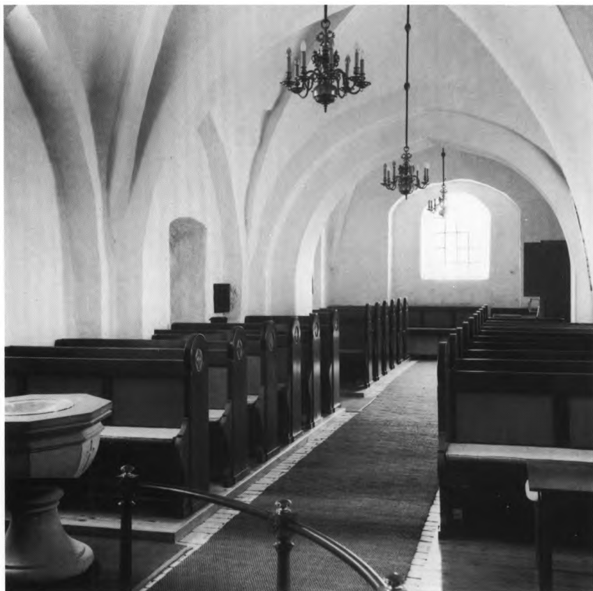
Fig. 10. Indre, set mod vest. NE fot. 1979. - Interior seen to the west.
