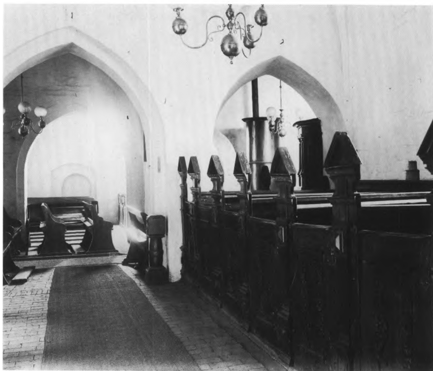
Fig. 35. Sydkapellets indre, set mod nord (s. 1125). Poul Nørlund fot. 1922. - Interior of the south chapel to the north.
