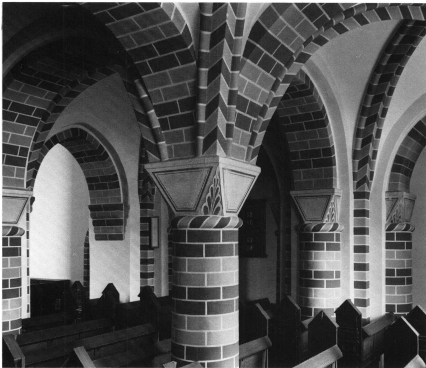
Fig. 16. Tårnrum, set mod sydøst (s. 1550). LL fot. 1980. - Tower chamber to the south-east.
