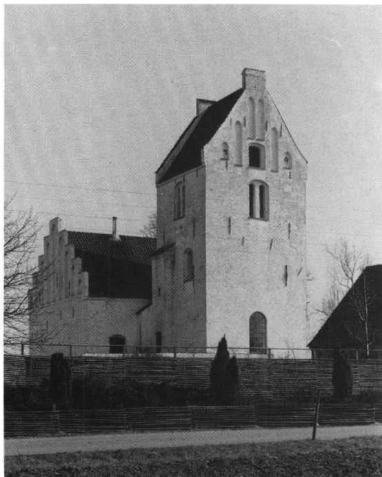
Fig. 6. Kirken, set fra nordvest. HJ fot. 1987. - The church seen from the north-west.
