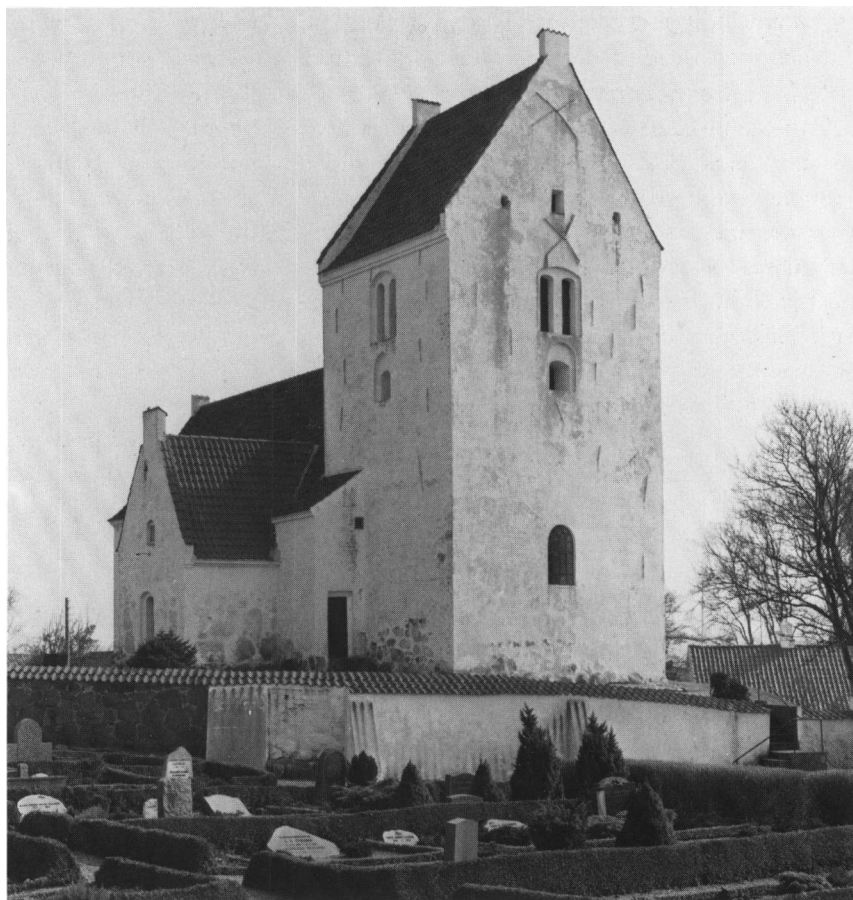
Fig. 3. Ydre, set fra nordvest. HJ fot. 1987. - Exterior seen from the north-west.
