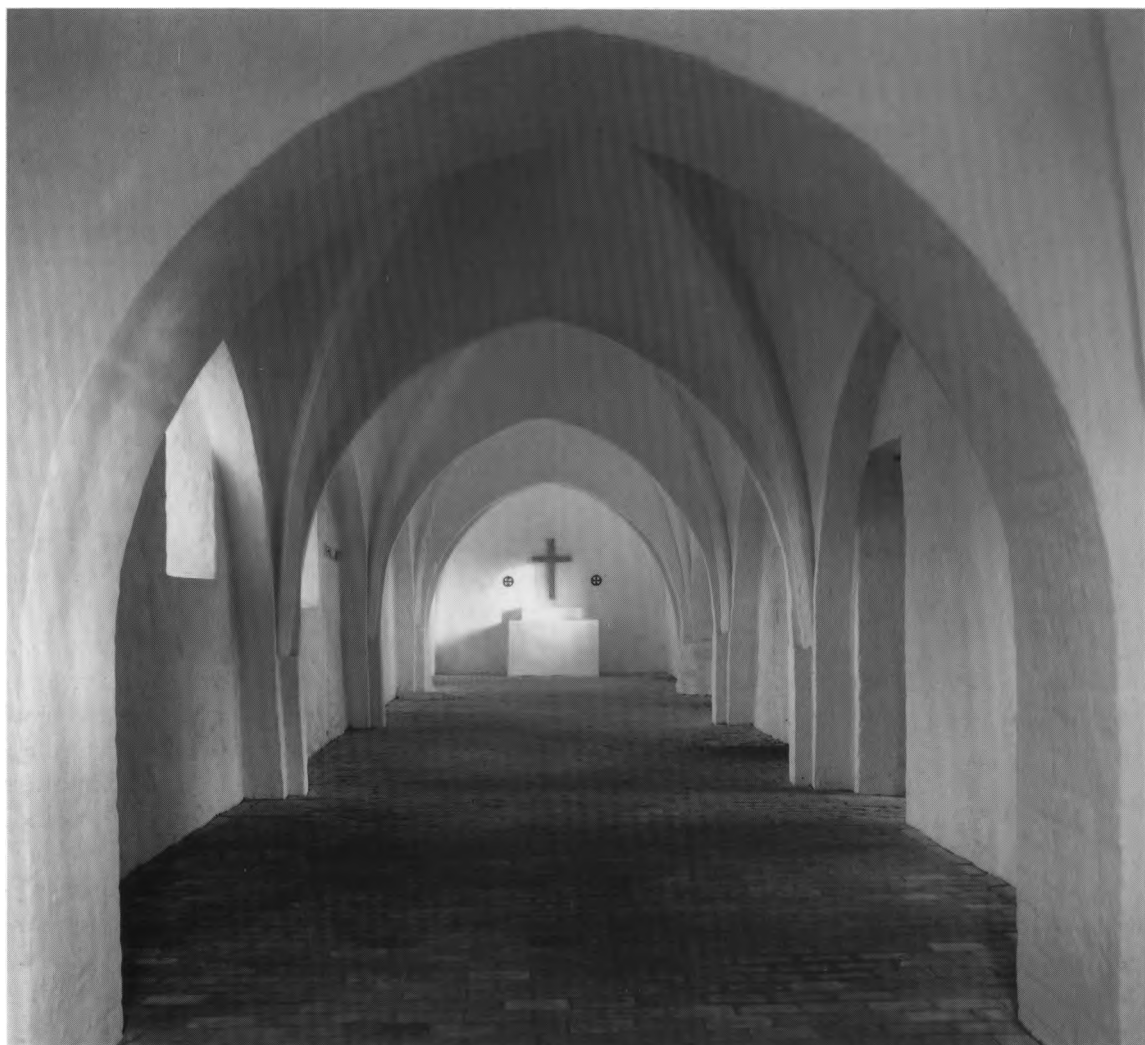
Fig. 6. Indre, set mod øst. NE fot. 1989. - Interior to the east.
