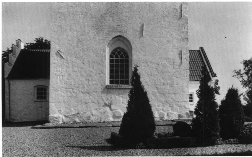
Fig. 8. Nedre del af tårnets vestfacade. Murværket er hovedsagelig af genanvendte sten fra kirkens oprindelige ttårn (s. 1931); dog stammer sydvesthjørnets kvadre fra en hovedreparation i 1600'ernes sidste årtier (s. 1932). HJ fot. 1989. - Lower part of the tower's west face. The masonry is principally re-used stone from the church's original tower; however the ashlar in the south-west corner are from a repair made at the close of the 17th century.
