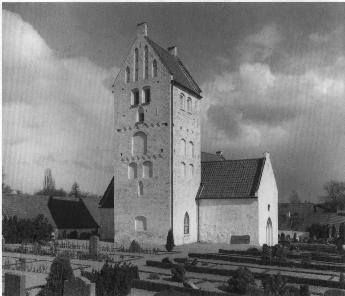
Fig. 6. Ydre, set fra sydvest. HJ fot. 1989. - Exterior seen from the south-west.
