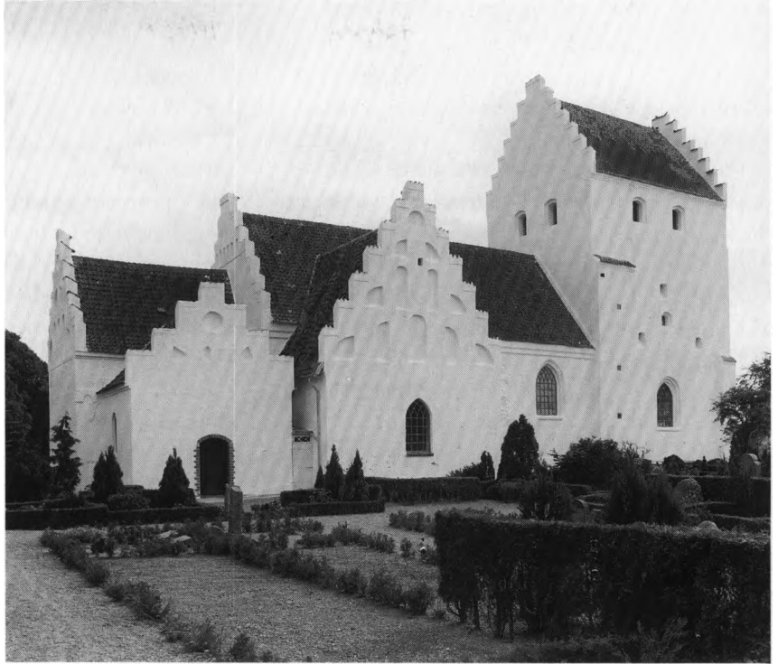
Fig.25. Kirken, set fra nord. NE fot. 1983. - Church seen from the north.
