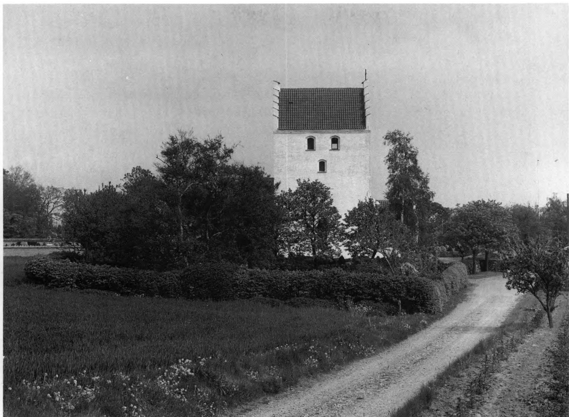
Fig.1. Ydre, set fra vest. NE fot. 1990. - Exterior seen from the west.
