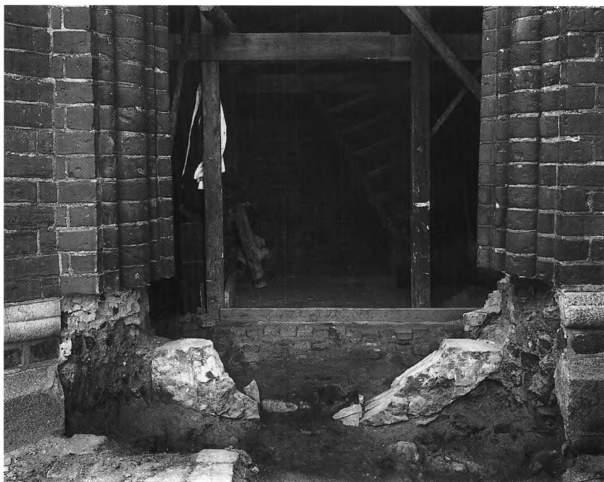
Fig. 68. Østportalens yderside under restaureringen 1917-21 (s. 3074). Mogens Clemmensens fot. - The external face of the east portal during the restoration of 1917-21.
