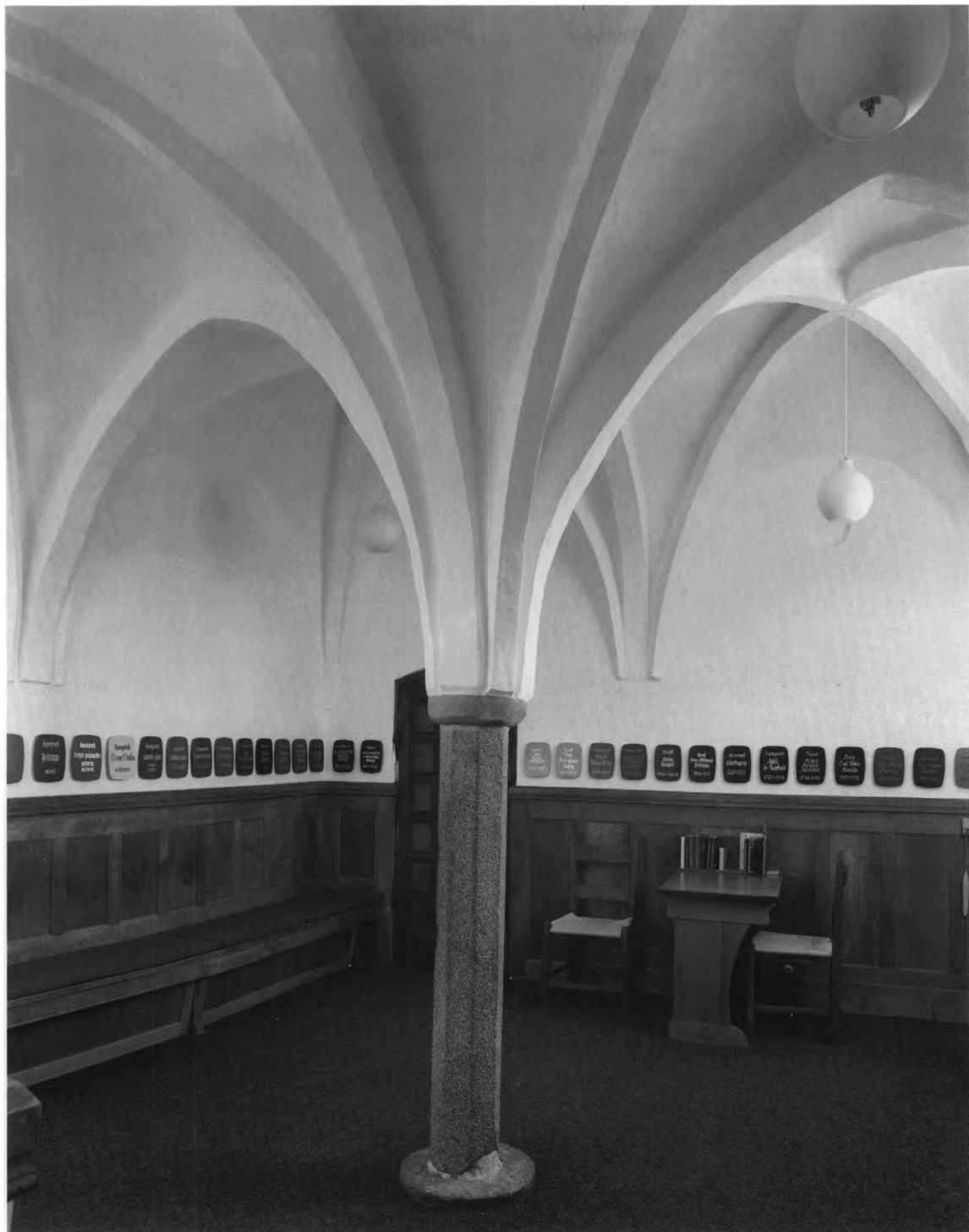
Fig. 106. Sakristiets søjlerum, set mod nordvest (s. 3104). NE fot. 1995. - Columned interior of the sacristy, seen to the north-west.
