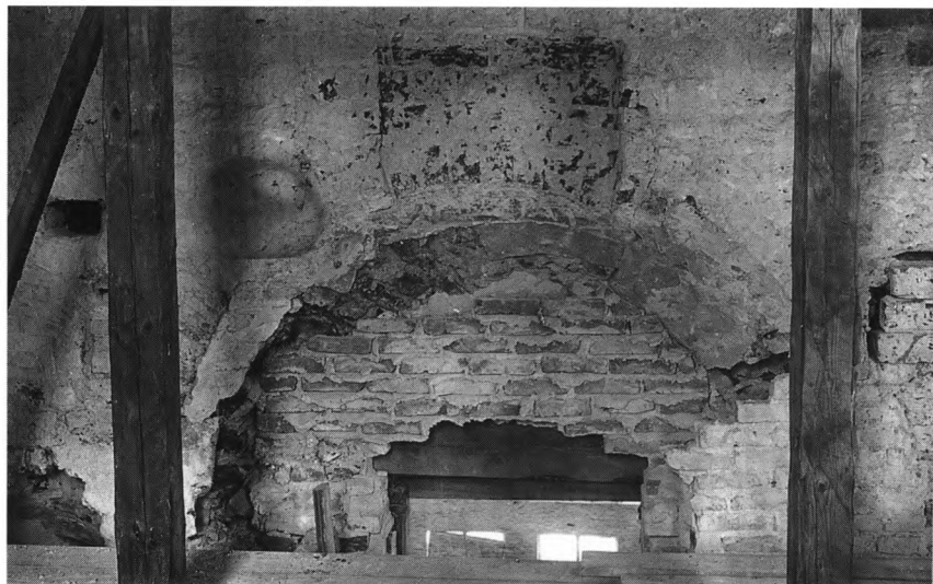
Fig. 67. Østportalens indre bueåbning under restaureringen 1917-21 (s. 3075). Mogens Clemmensens fot. - The east portal's interior arch during the restoration of 1917-21.
