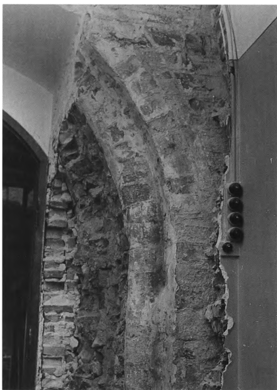
Fig. 12. Skibets syddør under fremdragning. EIM fot. 1957. - The south door of the nave is exposed.
