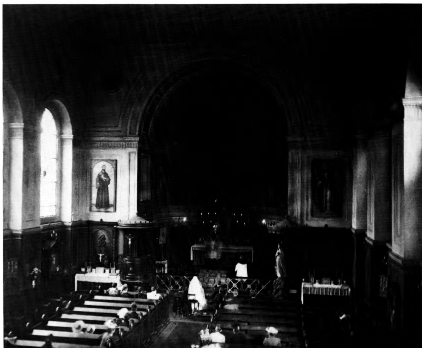
Fig. 119. Interiør mod øst. Ældre fot. mellem 1895 og 1898 (s. 432). KglBibl. — Interior to the east. Early photograph taken between 1895 and 1898.
