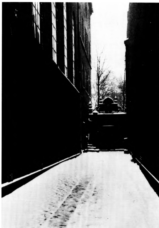
Fig. 60. Søndre sidegård med nu nedrevet portal mod haven (s. 366). Johs. Hoffmann fot. 1908. KglBibl. — South side-building with door (now demolished) into the garden, photograph 1908.
