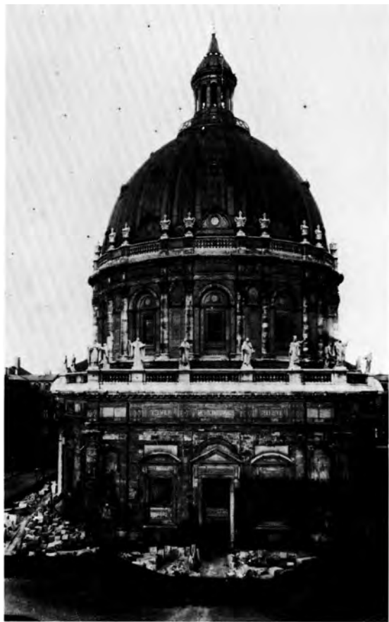
Fig. 287. Bagpartiet efter fjernelse af stilladset 1891. Kopier af Johannes Døberens og Elias' statuer er prøveopstillet foran facaden. Fot. KglBibl. – The rear of the building after the removal of scaffolding 1891. Copies of the statues of John the Baptist and Elijah in trial positions in front of the facade.
