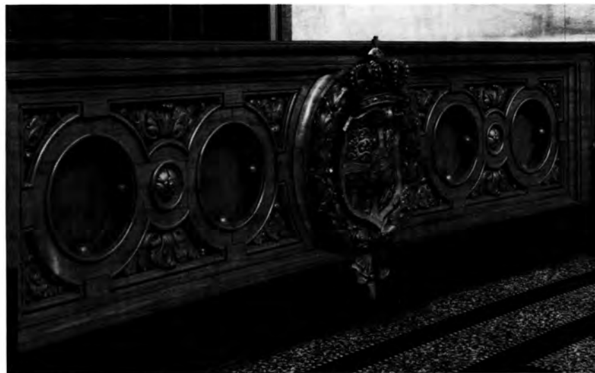
Fig. 264. Skranke ved kongestol (s. 747). LL fot. 1980. - Rail in front of the King's Pew.
