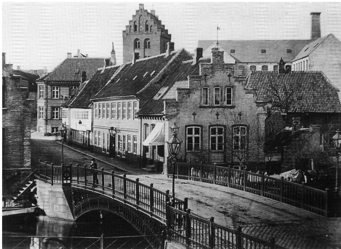
Fig. 5. Kirkens tårn, set fra syd. I forgrunden Frederiksbroen fra 1844, landets ældste vejbro af støbejern. Den høje bygning øst for kirkens tårn er Dorchs fabrik fra 1879, senere indrettet til Teknisk Skole og nu sognehus samt almennyttig beboelse (s. 1023). Ældre fot. o. 1880. - The church tower seen from the south. In the foreground Denmark's oldest cast-iron road bridge, Frederiksbroen, built in 1844. The tall building east of the church tower is Dorch's factory from 1819, later turned into the Technical College, and now the parish hall and community housing.
