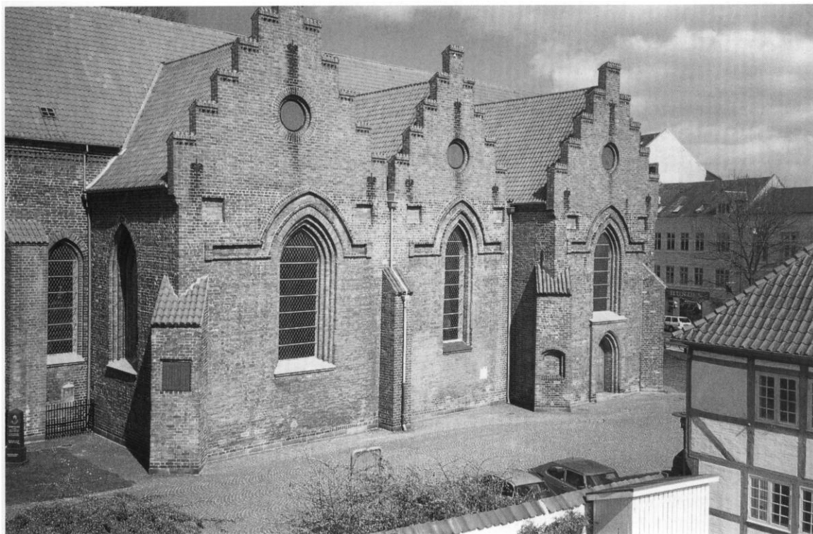
Fig. 331. Søndre sideskibs gavle, set fra sydvest. HJ fot. 1999. - Gables of the south side aisle, seen from the south-west.
