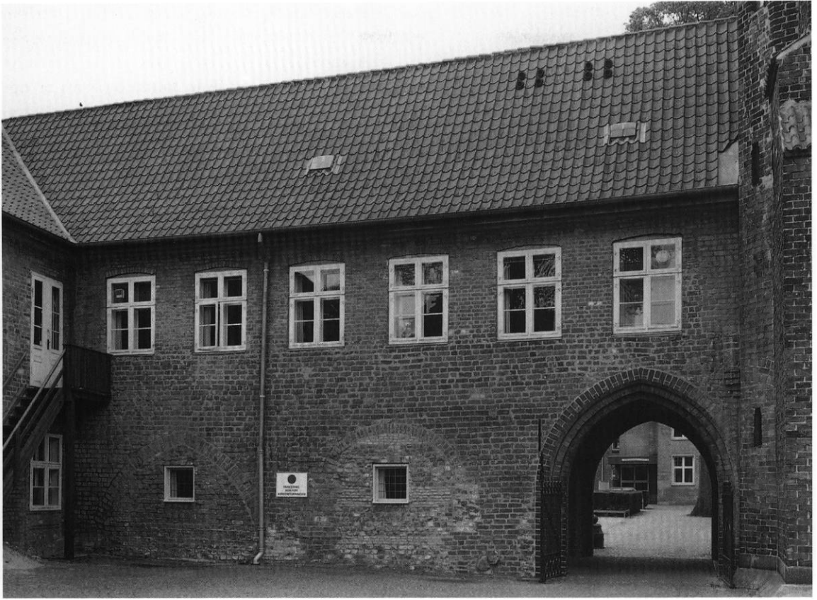
Fig. 93. Løngangen mellem kirke og slot, set fra syd (s. 1314f.). Henrik Wichmann fot. 1999. - Communication gallery between the church and castle seen from the south.
