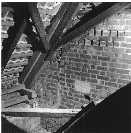
Fig. 309. Udsnit af midtskibets søndre overmur, set fra loftet over søndre sideskibs 3. fag. Gesimsens savskifter skæres af tagspor, hidrørende fra kapellernes lave tag, opsat 1748-50 (s. 1323). Savskifternes østre afslutning viser, at de har fulgt den vestre tagflade af et laveresiddende sadeltag, tilhørende sydkapellets vestre fag i dets oprindelige skikkelse (s. 1278). HJ fot. 1997. - Detail of the nave's south upper wall seen from the loft above the third bay of the south side aisle. The saw-tooth courses of the cornice are interrupted by roof traces from the chapels' low roofs put up in 1748-50. The east ends of the saw-tooth courses reveal that these courses followed the west roof surface of a lower pitched roof belonging to the west bay of the south chapel in its original form.
