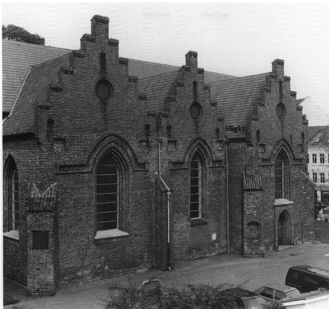
Fig. 85. Søndre sideskibs gavle, set fra sydvest. Henrik Wichmann fot. 1999. - Gables of the south side aisle, seen from the south-west.
