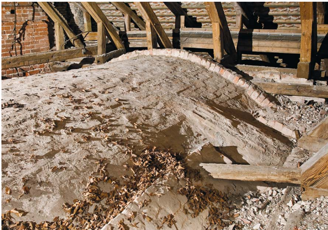
Fig. 34. Oversiden af søndre korsarms hvælv, set fra nordøst (s. 2128). Foto Arnold Mikkelsen 2008. – Upper side of the vaulting in the south transept, seen from the north-east.
