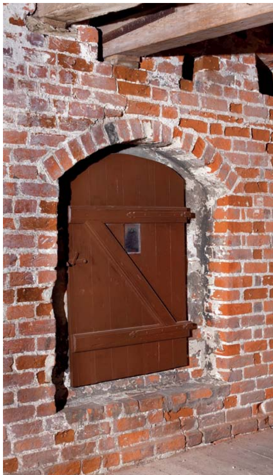
Fig. 35. Østre glåmhul i nordmuren i tårnets klokkestokværk, set fra sydvest (s. 2261). Foto Arnold Mikelsen 2009. – Eastern belfry light in the north wall of the bell-storey of the tower, seen from the southwest.
