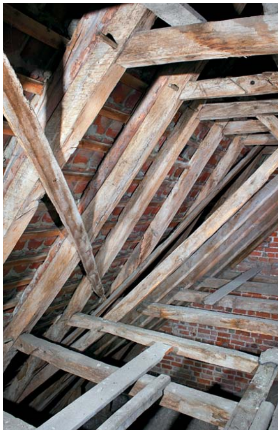
Fig. 66. Korsarmens tagværk (s. 2284), set fra nord. Foto Arnold Mikkelsen 2009. – Roof construction of the transept, seen from the north.
