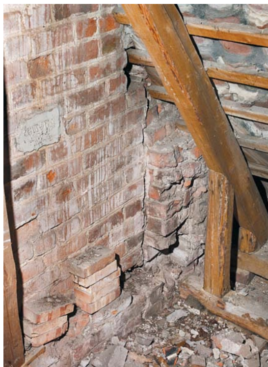
Fig. 48. Sammenstødet mellem midtskibets søndre arkademur og den søndre del af det teglsatte romanske \dagger skibs behuggede østgavl, set fra korsarmsloftet fra sydvest. Foto Arnold Mikkelsen 2010. – Junction between the south arcade wall of the nave and the south part of the east gable of the brick-built Romanesque \dagger nave, with treated surface, seen from the loft of the transept, from the southwest.
