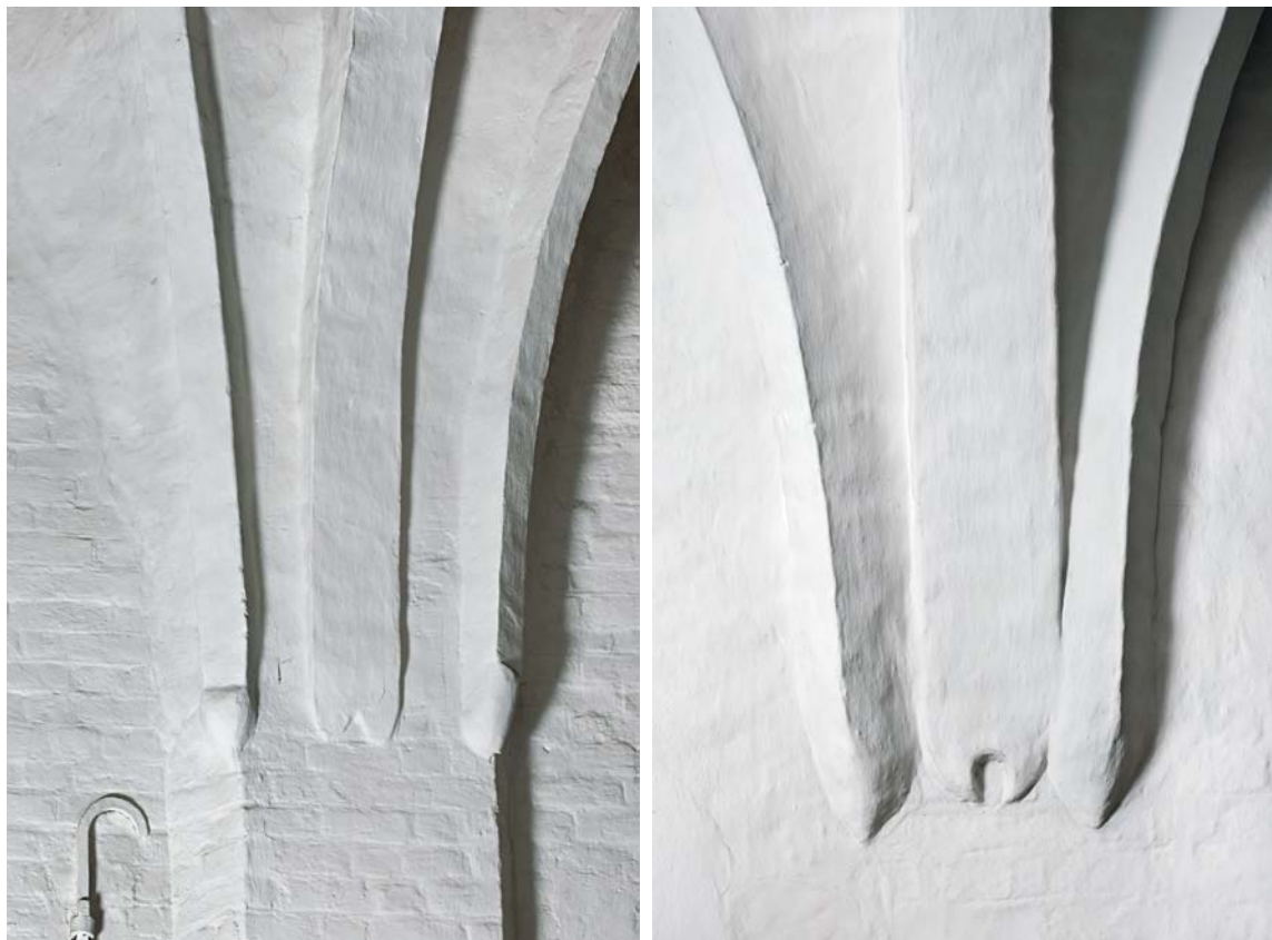
Fig. 54-55. Gjordbuekonsoller (s. 2277). 54. Mellem midtskibets to midterste hvælvfag, set fra syd. 55. Mellem søndre sideskibs to østligste hvælvfag, set fra nord. Foto Arnold Mikkelsen 2010. — Corbels. 54. The rib between the two central vault-sections of the nave, seen from the south. 55. The rib between the two eastern vault-sections of the south aisle.
