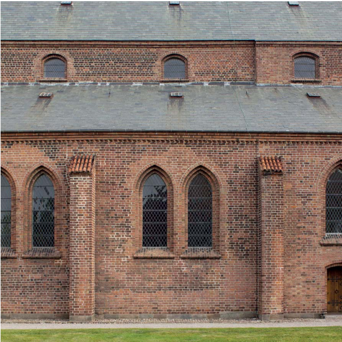
Fig. 27. Søndre sideskibs 5. fag fra øst, set fra syd (s. 2452 ff.). Foto Thomas Bertelsen 2011. – 5th bay from the east of the south side aisle, seen from the south.
