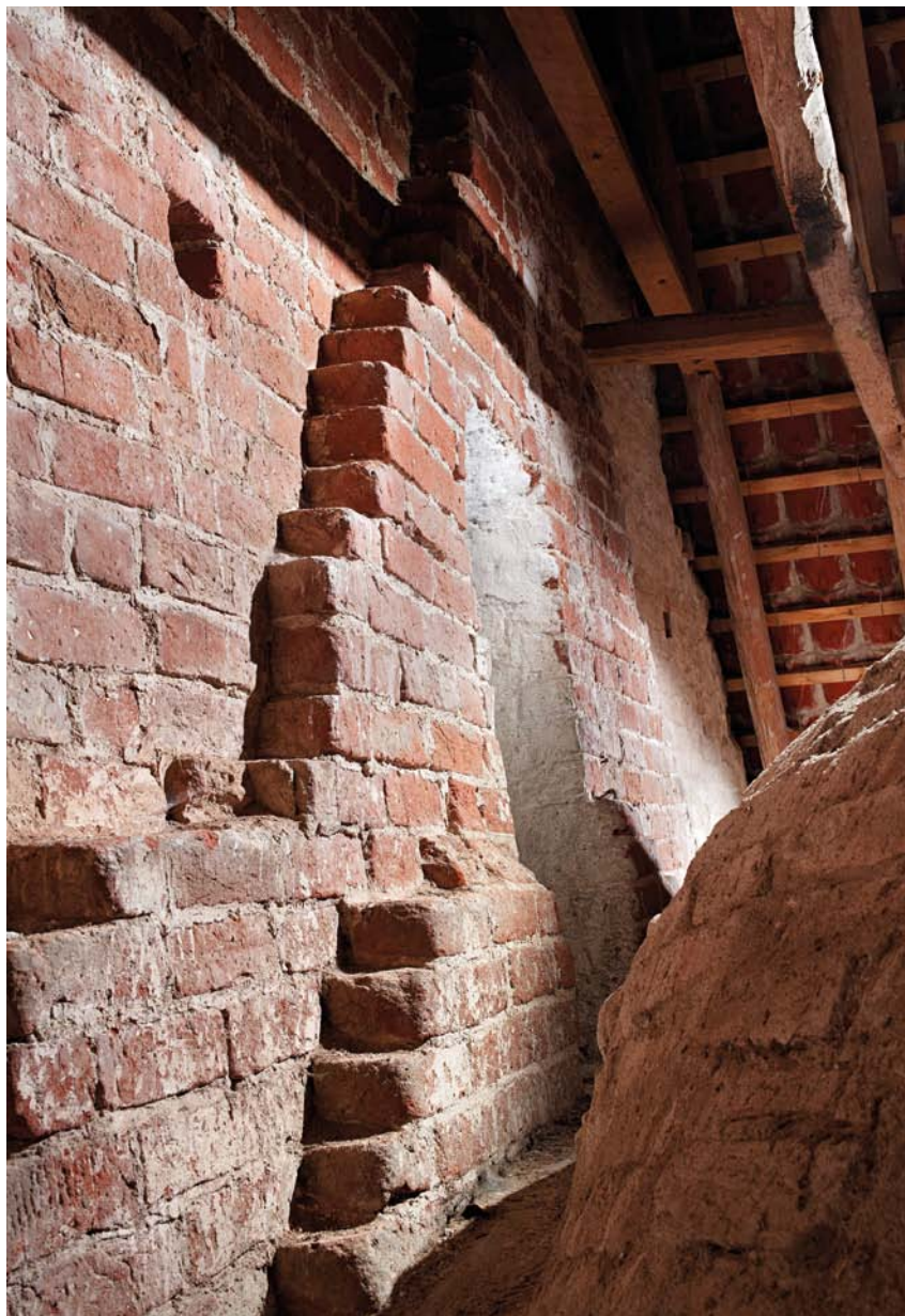
Fig. 12. Korets gotiske gavltrekant, integreret i den sengotiske østmur (s. 2650 og 2660), set over hvælvet mod øst. Foto Arnold Mikkelsen 2012. The Gothic triangular gable of the chancel, now integrated into the late Gothic east wall, seen towards the east from above the vault.
