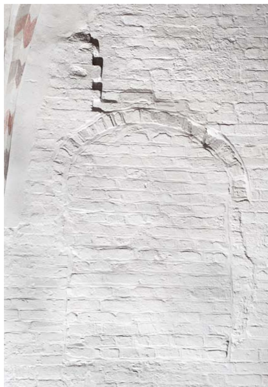
Fig. 95. Fortandingen mellem 1. og 2. byggefase i skibets sydvæg (s. 2799) umiddelbart vest for triumfmuren. Under fortandingen ses det blændede vindue, der har givet lys til prædikestolen (s. 2832). Foto Arnold Mikkelsen 2013. – Toothings between the 1st and 2nd building phase on the south-wall of the nave immediately to the west of the chancel arch wall. Beneath the toothings the bricked-up window which gave light to the pulpit can be seen.
