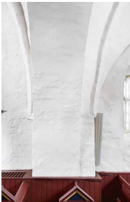
Fig. 6. Hvælvpille i langhusets nordside mellem 2. og 3. fag (s. 3278). Foto Arnold Mikkelsen 2014. – Vault pillar on north side of nave between 2nd and 3rd bay.
