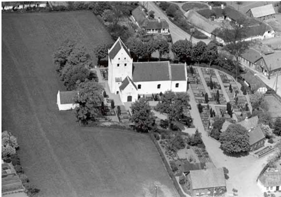
Fig. 2. Luftfoto af kirken og kirkegården set fra syd. Foto Sylvest Jensen 1939. I KglBibl. – Aerial photo of the church and churchyard seen from the south.
