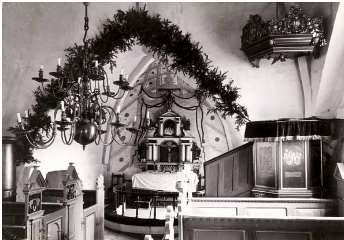
Fig. 82. Interior mod øst. Foto Kristian Hude 1903. – Interior looking east.
