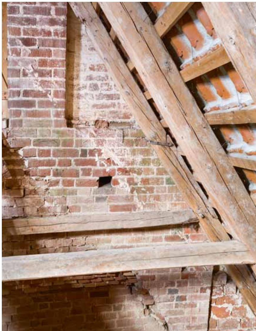
Fig. 32. Det romanske skibs vestgavls indre (s. 3705) med tagspor og tilmuret blænding i tårnets østmur (s. 3711), set mod vest. Foto Arnold Mikkelsen 2016. – Inside of west gable of Romanesque nave with roofing traces and bricked-up recess in east wall of tower, looking west.
