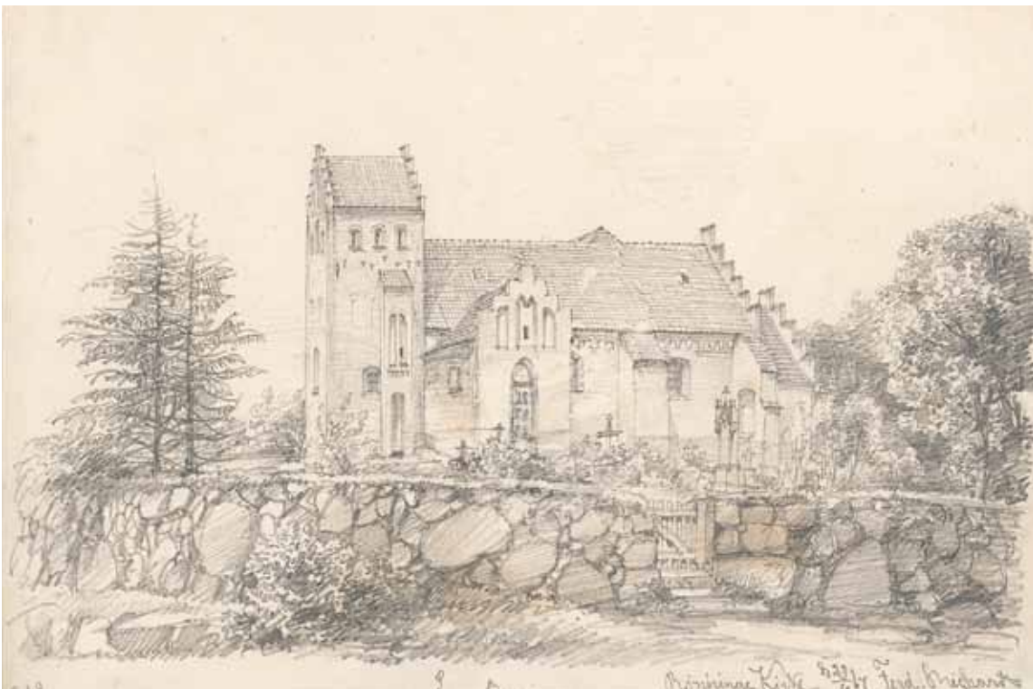
Fig. 4. Kirken set fra syd. Blyantstegning ved Ferdinand Richardt 1867. – The church seen from the south.
