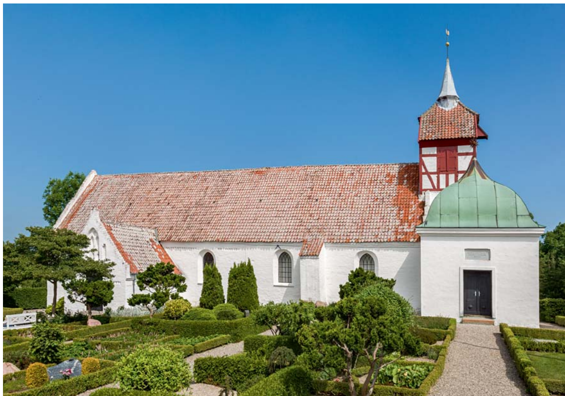
Fig. 1. Kirken set fra syd. Foto Arnold Mikkelsen 2017. – The church seen from the south.
