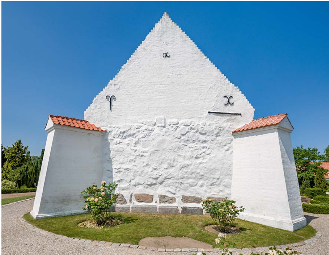
Fig. 11. Korets gavl (s. 4668) set fra øst. Foto Arnold Mikkelsen 2017. – The gable of the chancel seen from the east.
