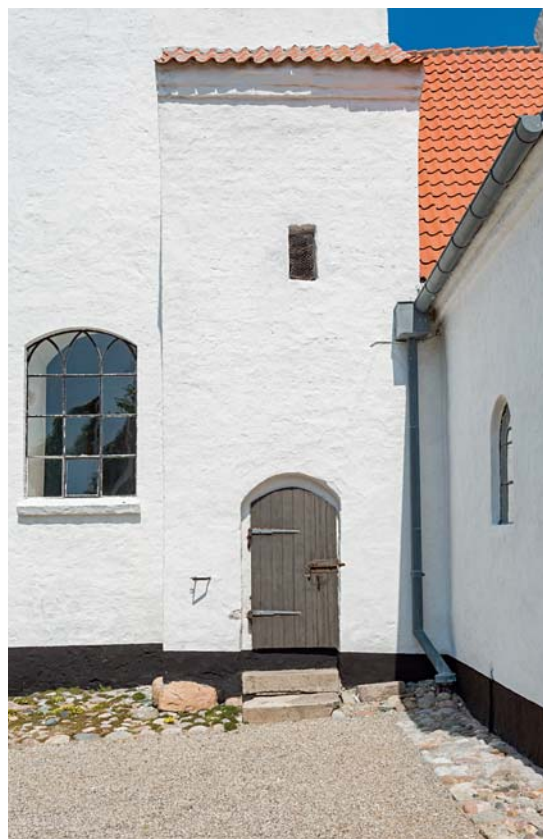
Fig. 69. Trappehus (s. 4738) set fra syd. Foto Arnold Mikkelsen 2017. – Stairwell seen from the south.
