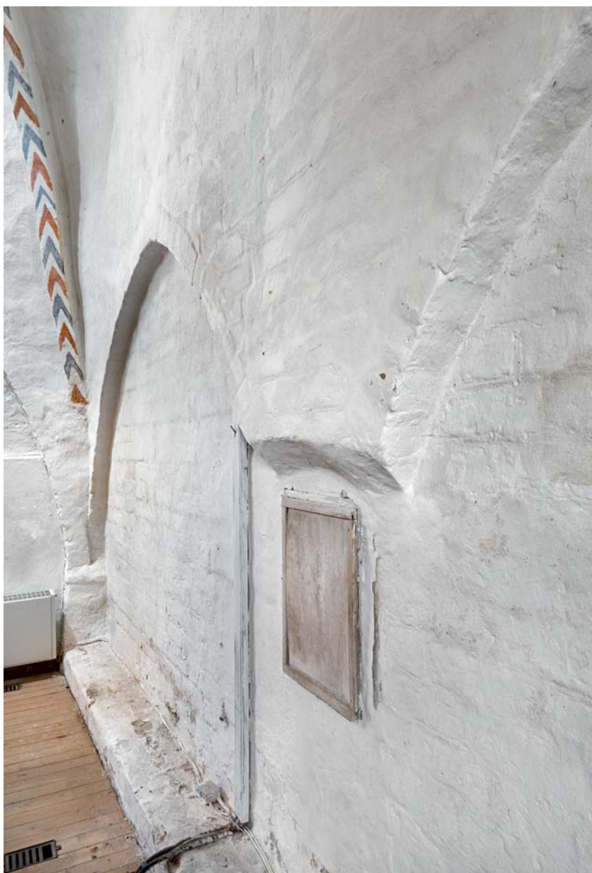
Fig. 8. Skjoldbuer i tårnets vestmur (s. 5175). Foto Arnold Mikkelsen 2018. – Wall ribs in the west wall of the tower.
