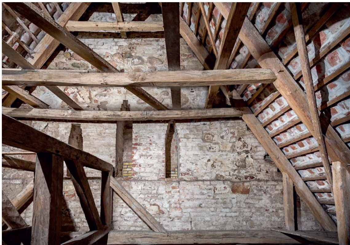
Fig. 13. Indersiden af de nu i facaden helt omdannede pibeformede åbninger i tårnets vestre gavltrekant (s. 5285). Foto Arnold Mikkelsen 2019. – Inside of the now converted in the facade pipe-shaped openings in the tower's western gable triangle.
